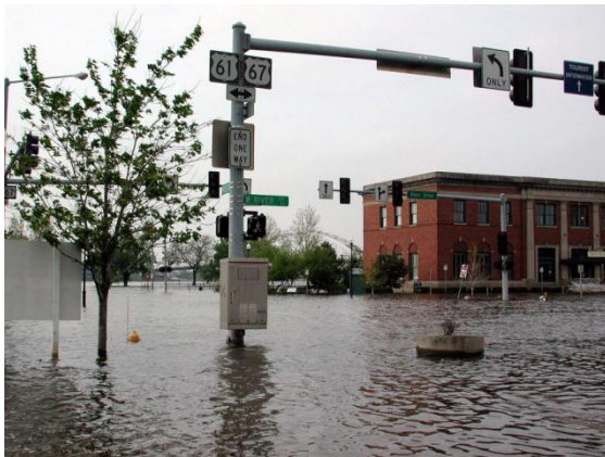
Flooding causes billions of dollars of damage each year. Flood maps provide only limited information. An on-site survey and assessment is needed to fully evaluate potential exposure and to identify mitigation opportunities.
